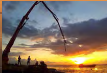
Hong Kong-Zhuhai-Macao Bridge
