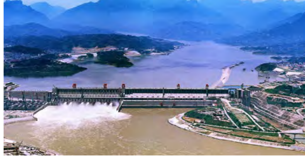
Three Gorges Dam, China
