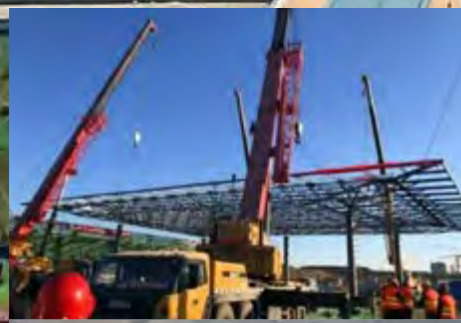
Beijing Daxing International Airport, China
